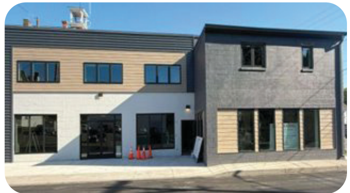
5 Chestnut St. in Geneseo after renovations
